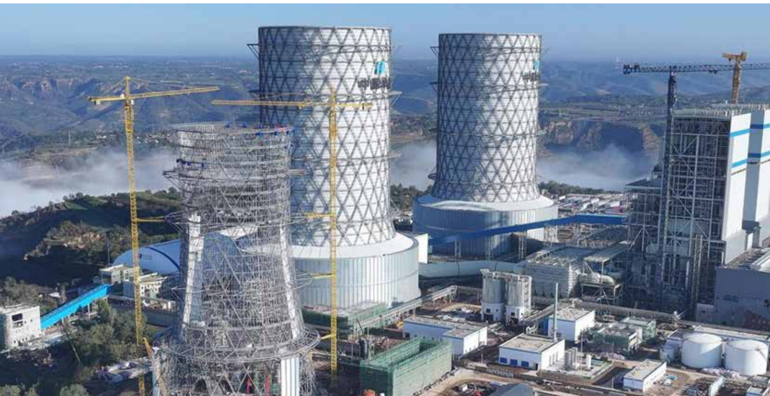
Longdong CCUS Project under construction
