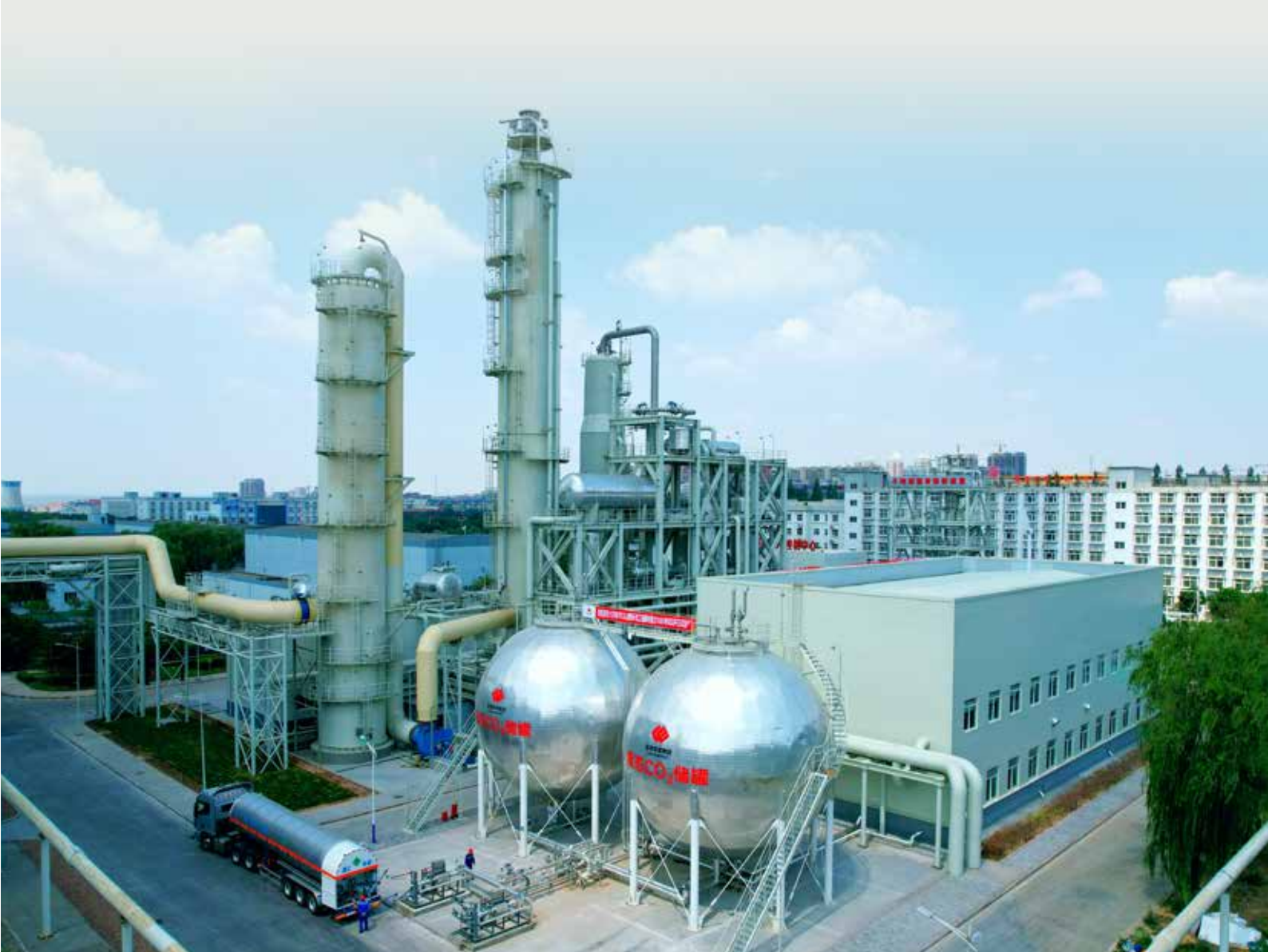
Figure 5: Jinjie 150,000 tpa CCUS demonstration project
