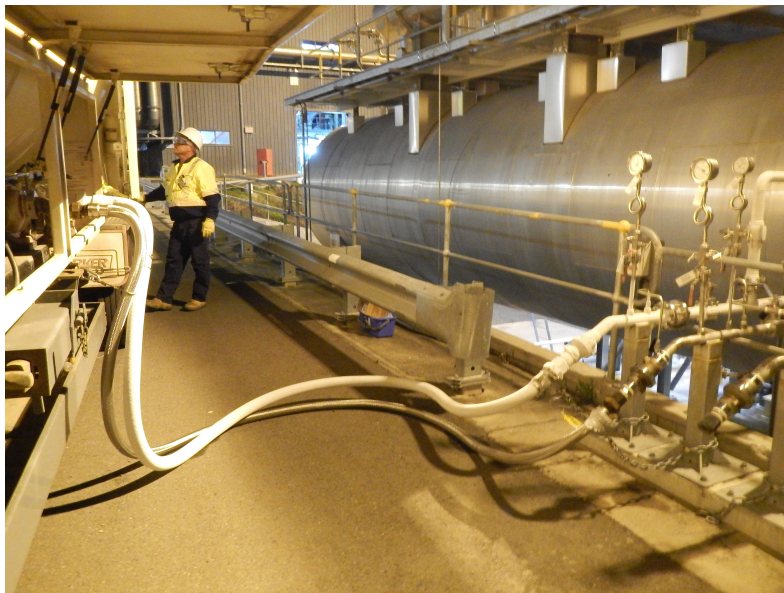
Figure 16 – Loading Liquid CO 2 into an Isotainer from the Callide A CO 2 storage tank (October 2014)
