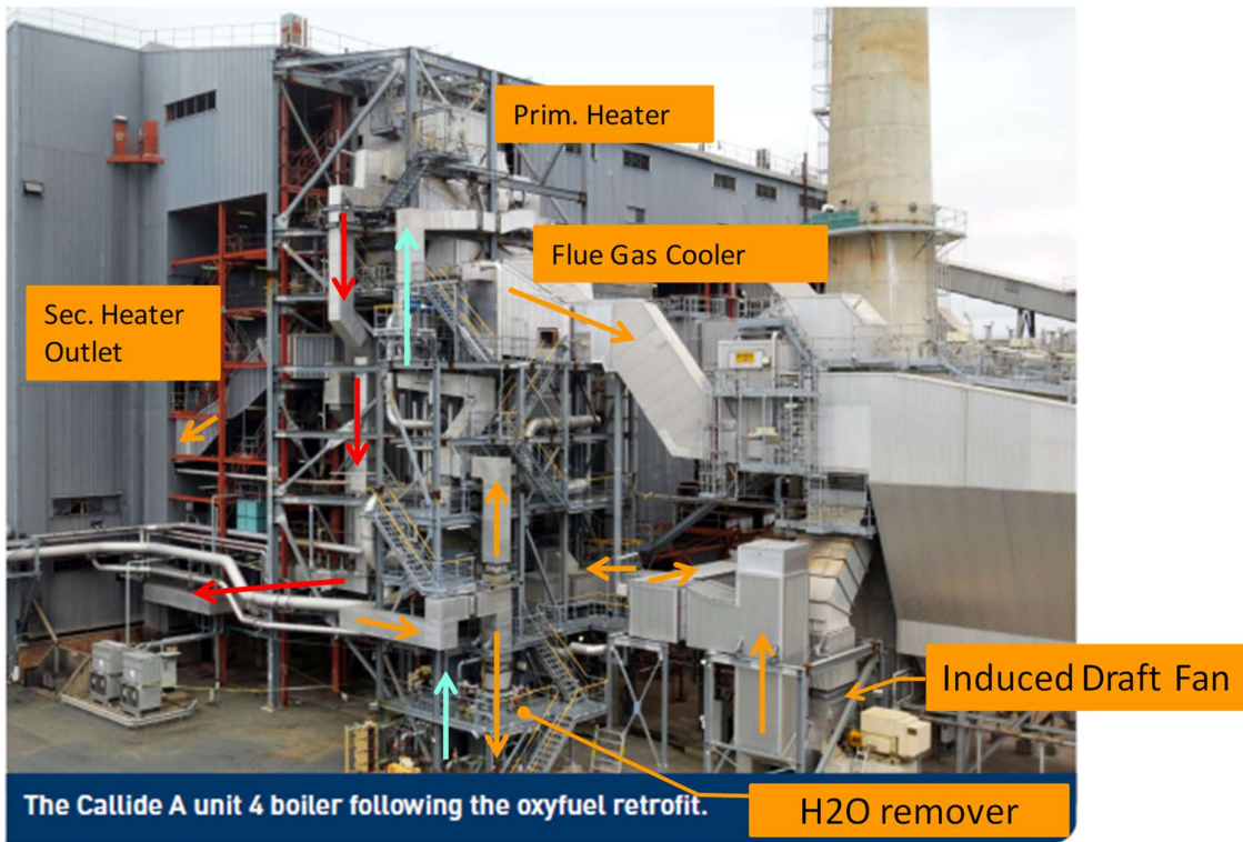
Figure 3 – Photo of Callide Oxyfuel boiler showing retrofit paths and flue gas flow directions
